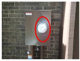
The 200-ampere, 120/240-volt electrical system enters the building via underground cables. The electric meter is located on the of the exterior building (see
