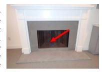
Due to the fireplace metal flue's configuration, our inspector was unable to evaluate its entire length. We recommend that you confirm the flue's condition, clearance and safety prior to using the fireplace.
