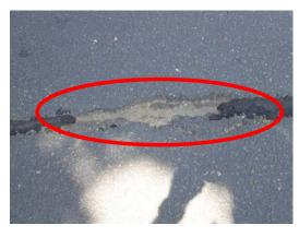
Portions of the "common" asphalt driveway surface and parking lot surface areas are starting to wear (see photos left and right for example areas). Filling the cracks with asphalt
