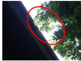
allowed to touch the exterior cladding or foundation or to obstruct a window view. Ideally, a minimum of twelve inches of clearance should be maintained between shrubs and exterior cladding and windows to prevent moisture from being trapped against the building structure, which may promote rot on and beneath vulnerable exterior components.
