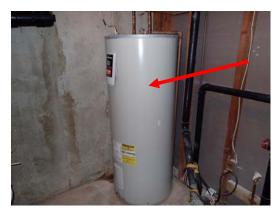
The water is heated by an independent, 80-gallon, electric, Bradford White brand, water heater (serial # AD4579698/ model #M280R6DS2 - see photo left) with a recovery rate of approximately 92 gallons per hour. The hot water supply system was evaluated and found to provide adequate amounts of hot water to all fixtures tested, at the time of this inspection.
